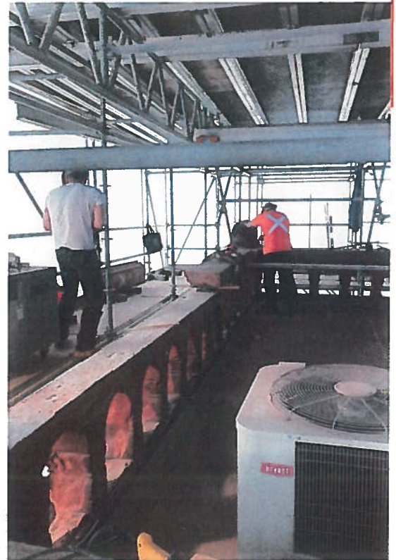
▲ Careful removal of damaged stonework. Photo The York Club, 2018
